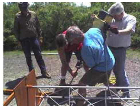
John, KB3XG and crew power driving tower stakes. With all that wind we lost no towers and stakes remained secure.
